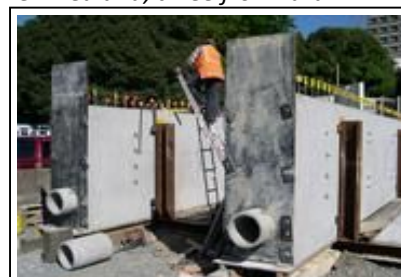
Stormwater treatment device construction, Auckland
