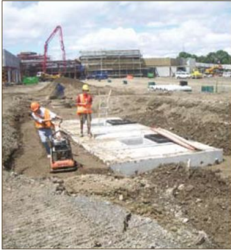
Installation of box-culvert StormFilter vaults
