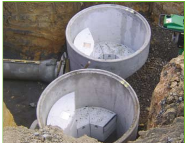
Installation of twin Hynds Up-Flo™ System
