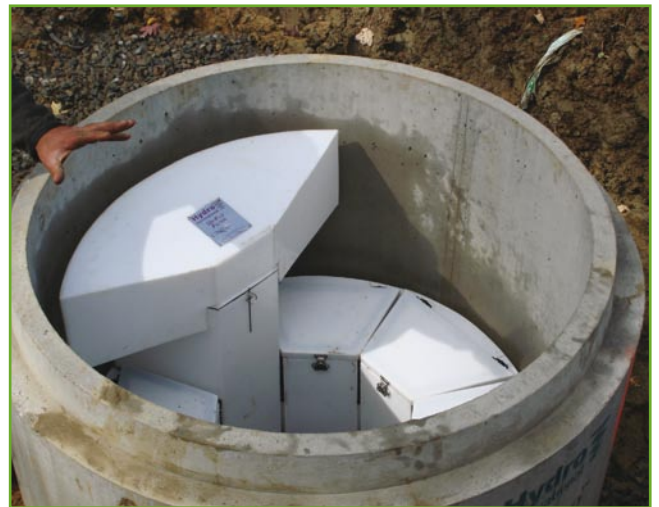
Installation of the Hynds Up-Flo™ Filter.
